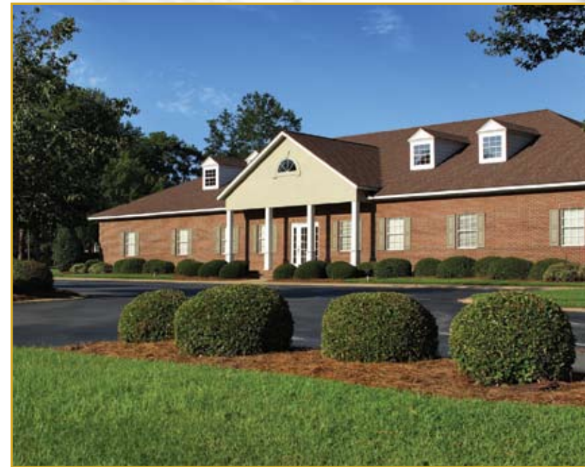
Valdosta Office: 2805 North Oak Street
